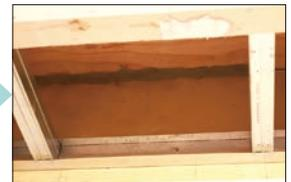
We filled the gap between the top of the parting wall and the flooring material of the second floor with fire-resistant putty. This eliminated the gap.
