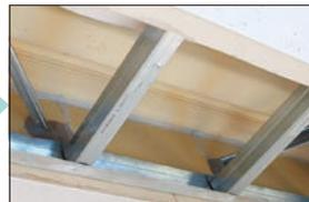
Gypsum boards was installed to serve as parting walls throughout the attic, and fire-resistant putty was used to prevent the gap in roofing material and beam. The corner-bracing joint was also filled with fire-resistant putty. Therefore, there remains no gap.
