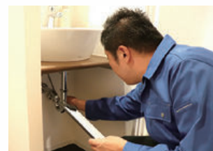
Management center staff carrying out an inspection
