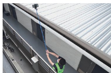
Building inspection in progress
