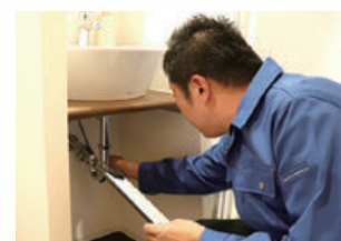
Management center staff carrying out an inspection
