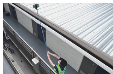
Building inspection in progress
