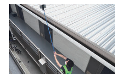
Building inspection in progress
